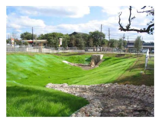
Figure 2: Example of Dry Detention Pond
