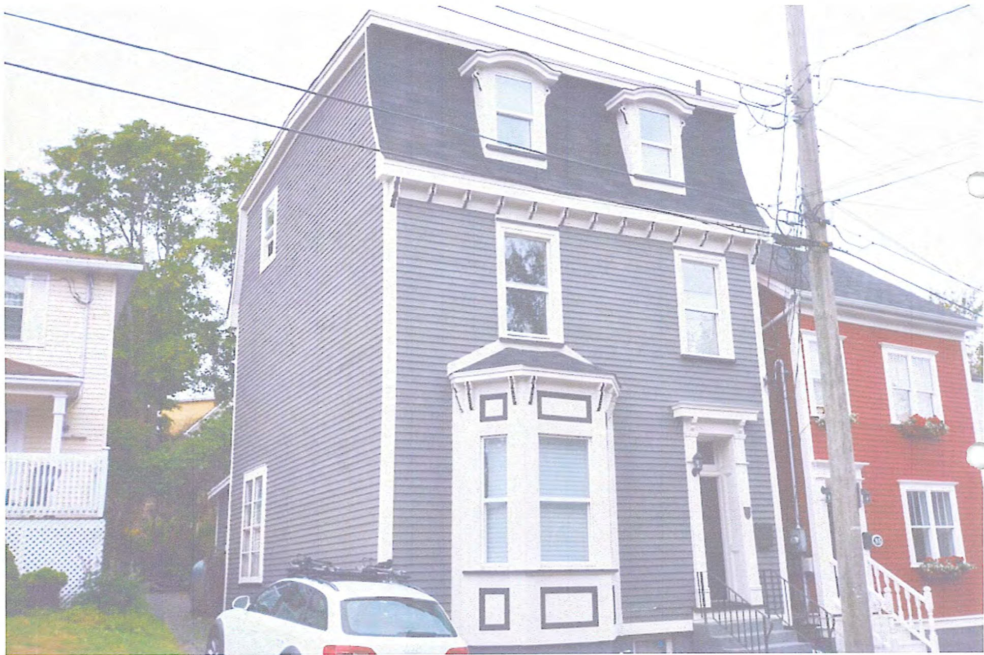
Current - photo after replacing exterior Clapboard, trim, windows, roof, insulation etc.
