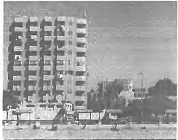
Fig. 1. The mobile phone base station antennas upon the building for agricultural professions.
