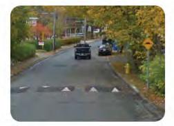
**VERTICAL**: A "bump" designed to make driving fast uncomfortable. Common tools include:
