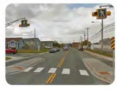
**HORIZONTAL**: Moving the edge of the driving lane to communicate a slower environment to drivers. Common tools include:
