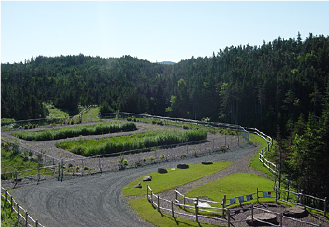
Photo 3: Abydoz System in Marystown, NL
