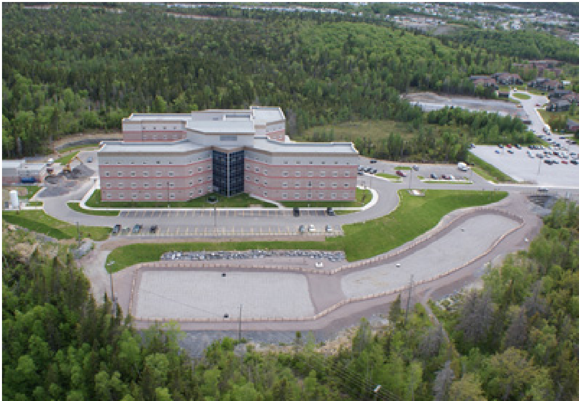
Photo 2: Abydoz System at the Long Term Care Facility in Corner Brook, NL
