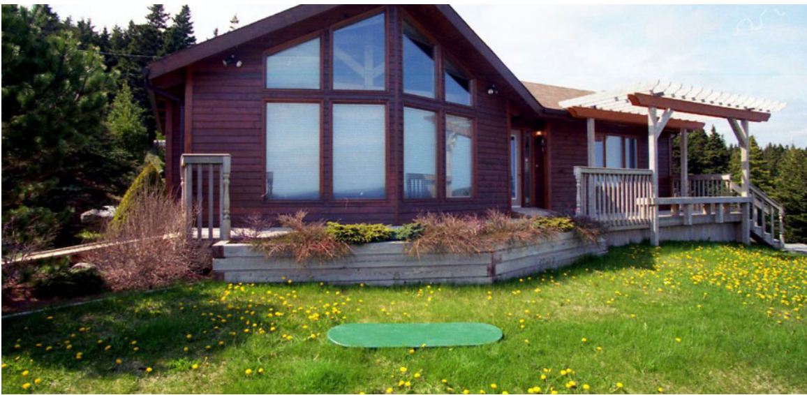
Photo 5: Below Grade Residential Clarity Biofilter System
