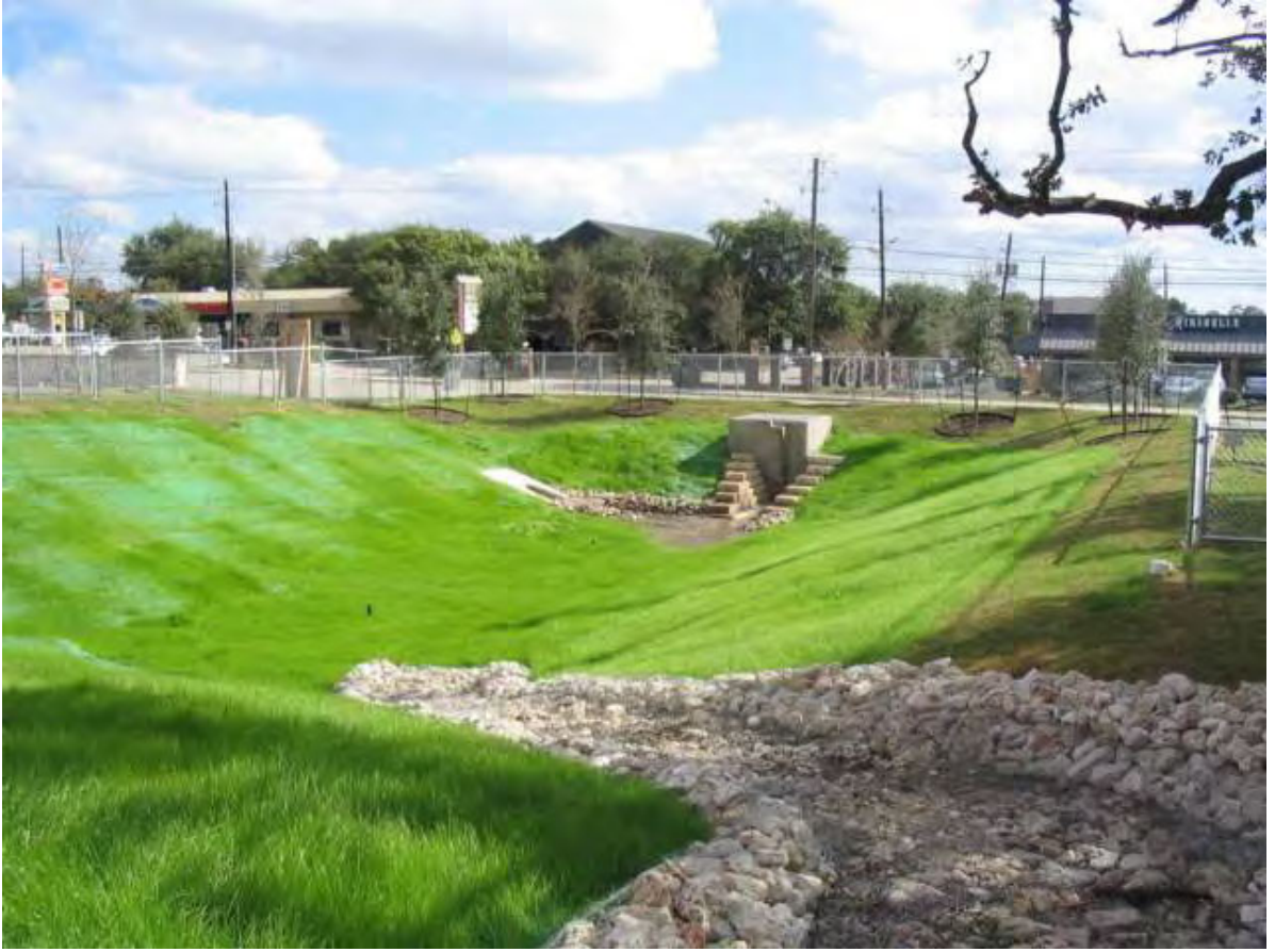
Figure 2: Example of Dry Detention Pond
