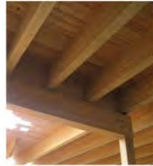
Glulam Beams & CLT deck
